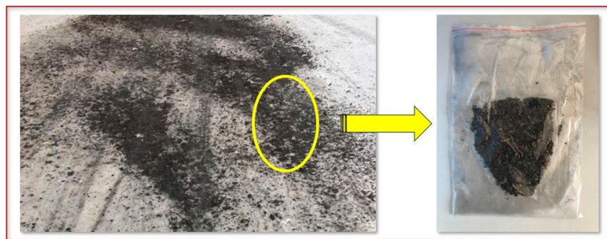
Figure 3. Anti-slip sand thrown on permeable pavement.
